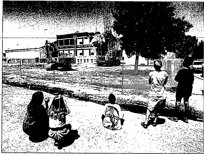
Demolition crews start pulverizing the old Hansen High School building Monday afternoon while residents like Jessica Reichel, Ashley Reichel, Mike Nelson, Jared Reichel and Tim Miller watch with an occasional 'Ooh' and 'Aah.'
