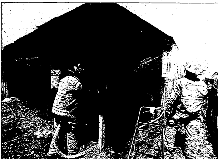
Twin Falls Fire Department Capt. Rick Frantz and Capt. Zeno Walker douse hot spots behind the wall of David and Mary Baunsgard's house at 1970 Poplar Ave., after a fire ravaged the structure Monday afternoon.
