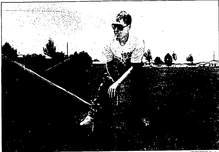
Emory Warren sets a sprinkler head in a playing field at Robert Stuart Junior High School in Twin Falls. Proposed increases in city water rates will cost local schools thousands of dollars.
