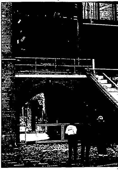
A bomb damaged Stockholm's Olympic Stadium Friday. No one was injured.
