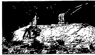
Workers clear off tarpaulin that had been covering a controversial mound of dirt at 408 Washington St. N. Monday afternoon before excavating the soil.
