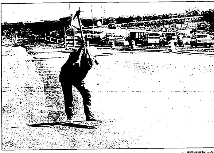
Victor Cantu works on the road surface of the new interchange on U.S. Highway 30 Tuesday. The Idaho Transportation Department has planned its work schedule to make sure traffic flows smoothly to the county fair in Filer.
