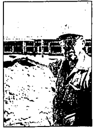
Fair Manager Dean Draper stands near an exposed sewer line that is being replaced after it gave out because of an unusual cloudburst and usual fair-time stresses.
