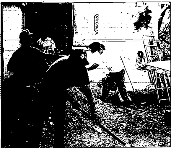
Roger England, left, Carl Gibbs and Tony Rost shovel debris from the foundation of an old pantry at the home of Judy Sirucek on East Main in Wendell recently. They are some of the volunteers helping to put Sirucek's home up to building code standards.
