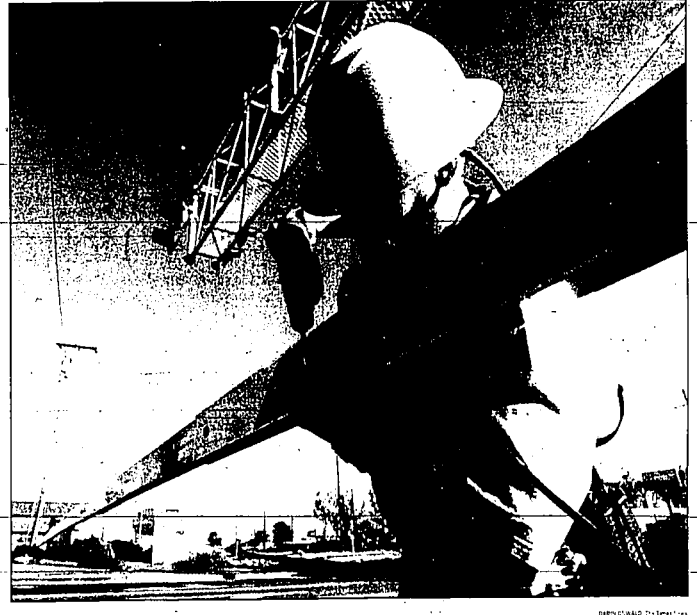
Paul Rodgers of Twin Falls replaces a railroad crossing arm at Blue Lakes Boulevard and Kimberly Road Monday afternoon. A truck shear cut the arm as it lowered earlier in the day.
