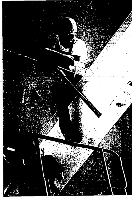
Marty Fugus attaches a support to the roof of the new $13 million manufacturing plant on Eastland Drive. The company, Clear Shield National, hopes production will begin in the new facility by March.
