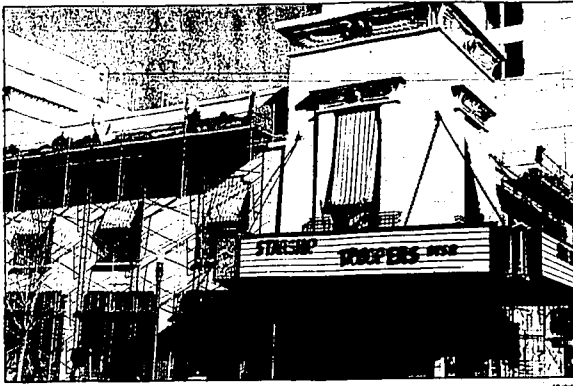
Scaffolding is up around Boise's Egyptian Theater to renovate part of the exterior, but state officials are alarmed about a leaky roof which is damaging the interior on the building, which is listed on the National Register of Historic Places.
