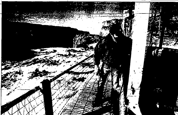
Dennis Bramon hooks and pulls up the large spill gates above Shoshone Falls. The gates are being lifted as higher flows come down the Snake River. DARRIN OSWALD/The Times-News
