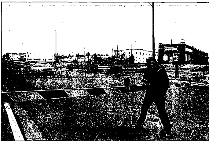
Signal maintenance worker Larry Shepherd repairs the lights on a railroad crossing arm on Oakley Avenue in Burley Wednesday afternoon.
