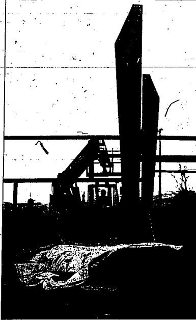
Workers ready the structure at what will be the Burley High School Theater Center for the roof, which is scheduled to be installed today.
