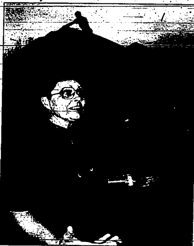
Rita Rouleau rethinks her reason for living in Florida as volunteer workers make the roof of her home at the Lakeside Estates community in Kissimmee Fla. Like many central Florida residents who relocated here for the year-round sunshine and healthy economy, the 53-year-old widow is having second thoughts after a tornado ripped apart her home a week ago.
