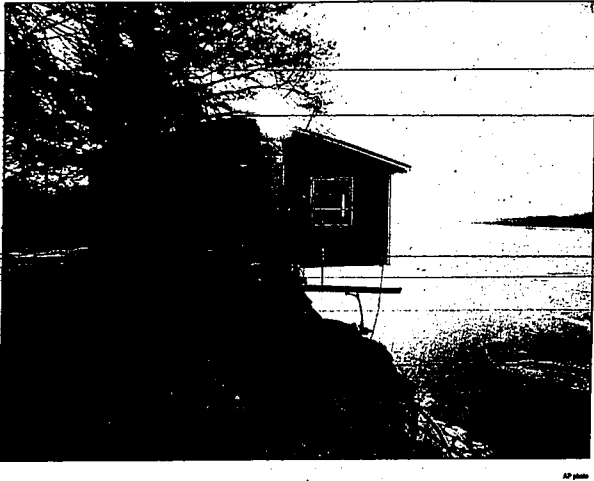
A house in the Twin Lakes community, near Crescent, Okla., hangs over the Cimarron River as the sun rises Wednesday. Heavy rains forced the river to change its channel and wash away land behind the house. Two houses have already been washed away from the community.
