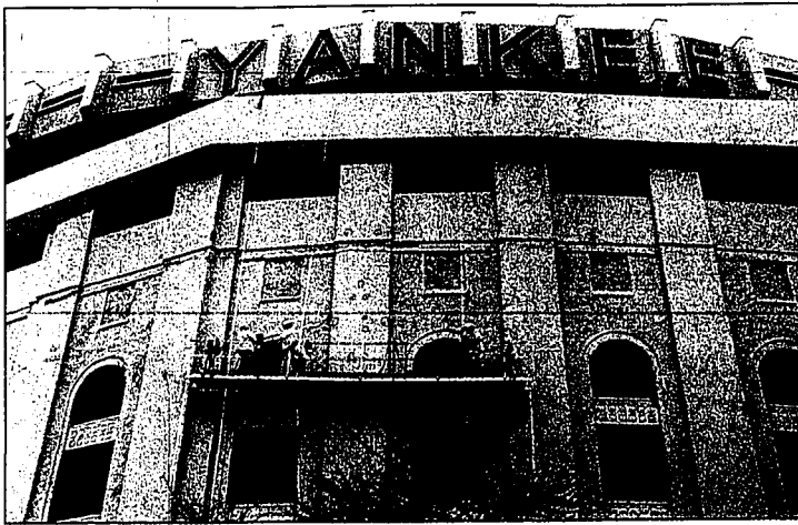
Workers repair Yankee Stadium's facade Friday in the New York borough of the Bronx. Work began Thursday to repair water damage to the concrete facade of the stadium, closed since a 500-pound steel-and-concrete joint fell and flattened seats in the stadium's mid-field deck on Monday.
