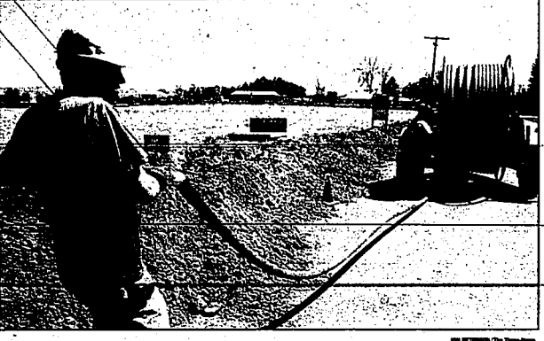
A worker with J.D. Dayley and Sons Construction lays the bright orange housing for fiber optic cable on A Street in Rupert Monday. The line will go to Declo, where Project Mutual Telephone and Albion Telephones are linking cable to give PWT an alternate route in and help Albion create a 'ring,' a loop of connections that will help the company keep lines open everywhere even when a section has been severed, said engineer Gary Earl. The Declo connection will also let the two companies swap cable television channels, he said.
