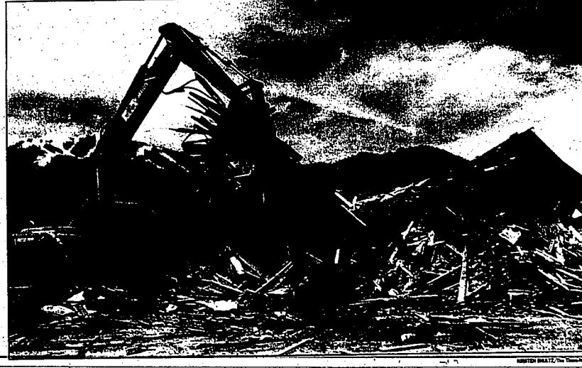
Excavation crews work to finish demolition of the old Colonnade building in Ketchum earlier this week. Rock from a casino hidden inside the building will be used for the site's new structure in June.
