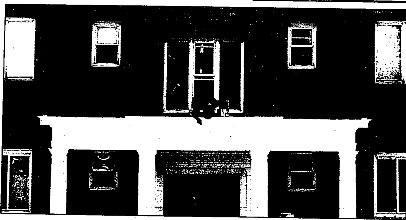
Parked above the entrance of Rax Arms Apartments on Sboosboe Street in Twin Falls, Steve Ewanluk brushes on a new coat of white paint.
