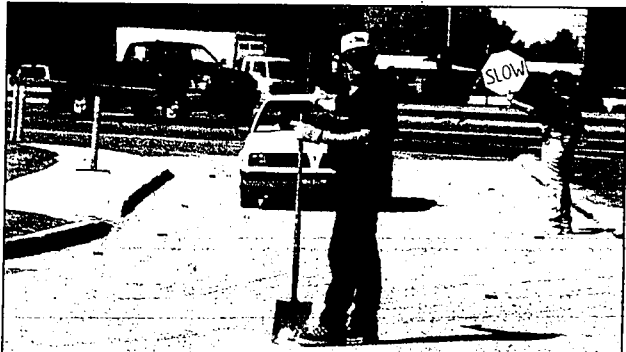
Construction workers hold up traffic at the intersection of Overland Avenue and North Fifth Street Thursday morning as Burley's Fifth Street surface gets a touch-up.
