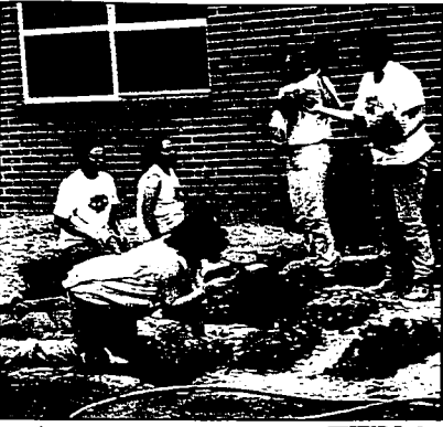
Members of the Maltz Job Training Partnership Act team finish some improvements at Raft River High School last week.
