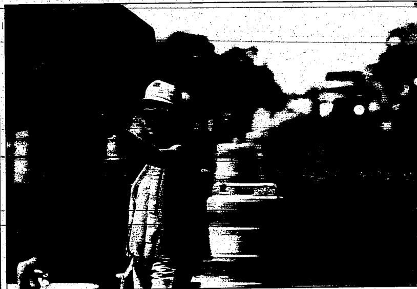
Trudy Whaley of Hansen directs traffic through the construction zone on Addison Avenue West. Hansen's crews are ready to repair the heavy stretch of road in Twin Falls.
