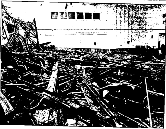
An overall view of the Universal Church of God building in Osasco, Brazil, where at least 30 people were killed and more than 500 injured when the roof collapsed during a late night vigil celebration Saturday. More than 1,500 people were gathered at the time. The building had been an old movie theater but was being used as a church.
