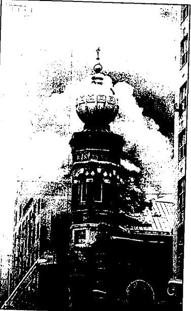
Smoke billows from a fire as it rips through the Central Synagogue in New York on Aug. 28. The Moorish-style synagogue, built between 1870 and 1872, is a city and national landmark.
