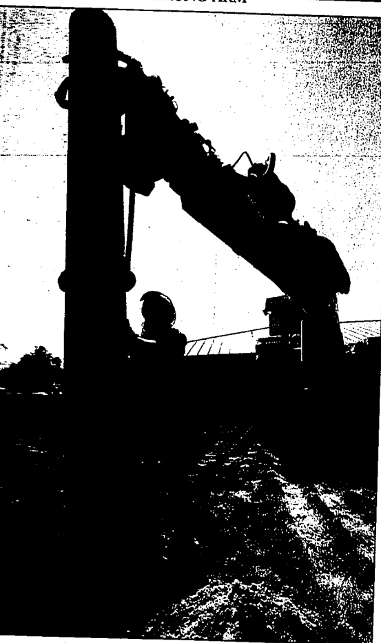
On Thursday night, a pole before putting it around the base to secure it. The pole used power poles. were placed in Canyon View Park, and Addition Services by Idaho Power and will be used for a "ropes course," to teach patients trust and teamwork.
