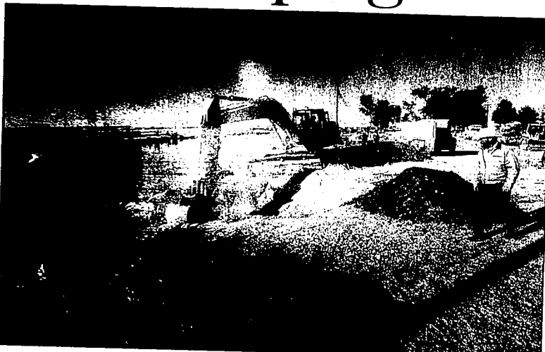
Workers work frantically to plug a 30-foot hole in an earthen levee at Milner Dam Thursday morning. A voluntary evacuation notice was issued for homes downstream, but was rescinded after the leak was sealed.
