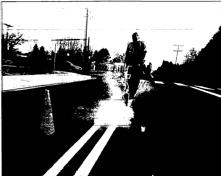
Liamer Gillette scrapes the center line off Filer Avenue in front of Twin Falls High School to paint a new line and make room for concrete dividers to be installed later.
