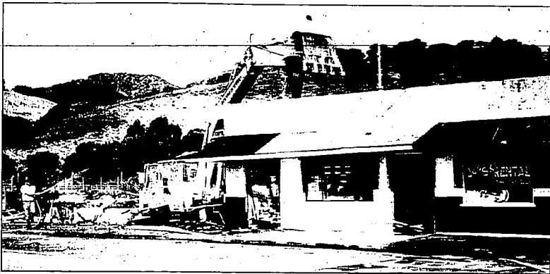
Demolition work begins Tuesday on a rental shop on the 500 block of Front Street in Avila Beach, Calif. The demolition marks the beginning of an 18-month cleanup project of 400,000 gallons of toxins beneath the popular central beach town 10 miles south of San Luis Obispo, Calif.
