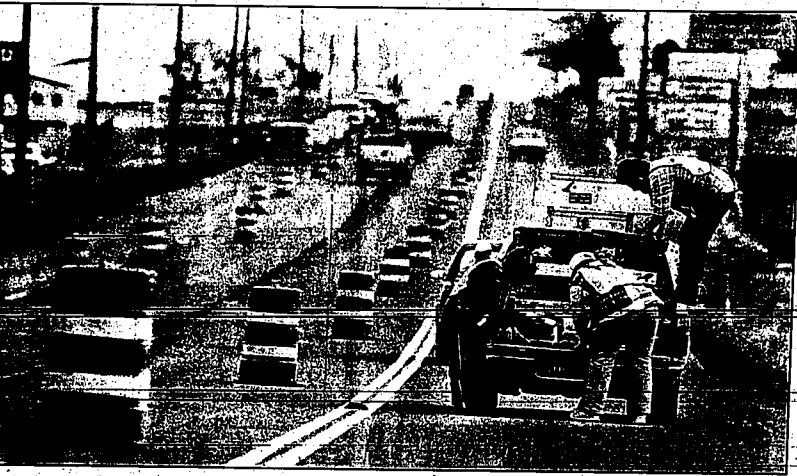
Road work on U.S. Highway 30 between Twin Falls and the Curry Junction at U.S. Highway 93 Monday. The $6.1 million project will widen the stretch of road to five lanes and is scheduled to be finished by November, the Idaho Transportation Department said in a news release.
