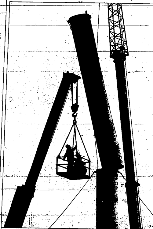
Mark Schelwie of Filer, working for Twin Falls Crane, is lowered away from an abandoned smokestack at Gooding's old tuberculosis hospital Monday. Schelwie had cut through the top section with a Newtron. The Idaho Department of Lands had ordered demolition of the 110-foot, 17,000-pound steel stack.
