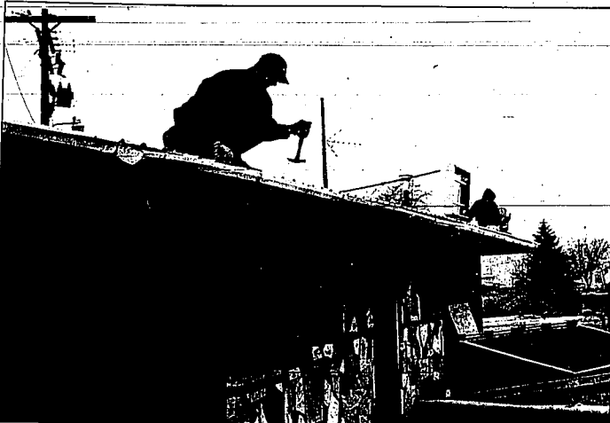
Jake Bowen, left, and Leland Johnson repair the roof at the new Silver Boot Saloon, formerly NIXX, in Dec. Thursday afternoon. Manager Randy Sparks said the new Southern rock/country Western saloon is scheduled to open by the beginning of March.
