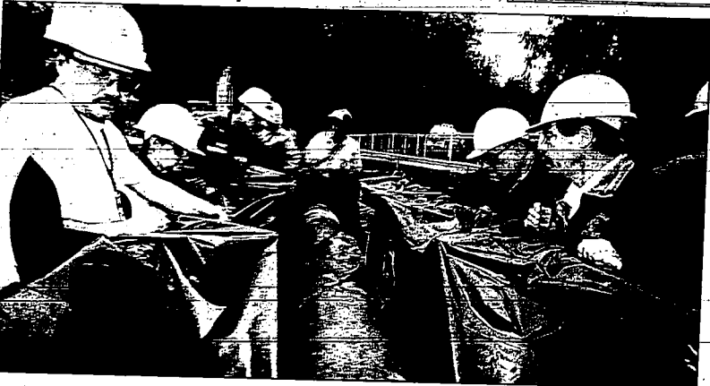
Workers examine a damaged section of pipe extracted Wednesday from the Olympic Pipe Line Co. fuel pipeline that exploded in Bellingham, Wash., June 20. The rupture in the pipe is said to be a key piece of evidence in the National Transportation Safety Board's investigation into the cause of the pipeline accident, that killed three youths and affected gasoline prices across the state.
