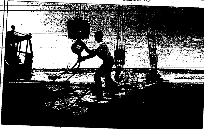
David Outler hooks a cable to a crane that will lift a 21-ton pipeline bridge over the High Line Canal south of Kimberly on Friday. The pipe had been buried under the canal but a leak forced the Twin Falls Canal Company to move the pipe.
