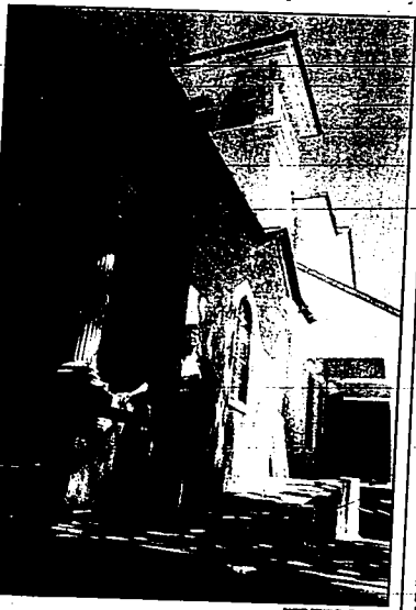
The Eighth Street Center, built in a Greek revival style, will house a variety of things including offices, building owner Kathy Ruyts said.
