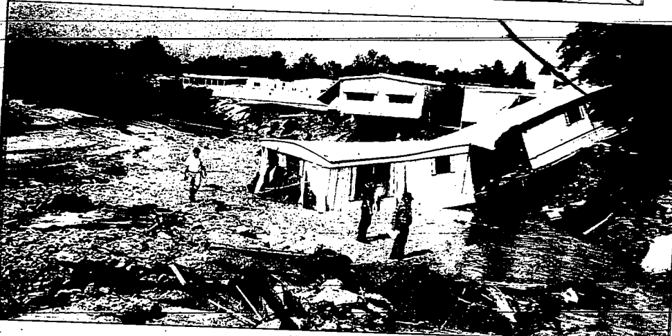
Clark County building inspectors investigate flood damage on the banks of the Flamingo Wash in Las Vegas Friday. Torrential rains on Thursday caused the worst flash flooding seen in 25 years.
