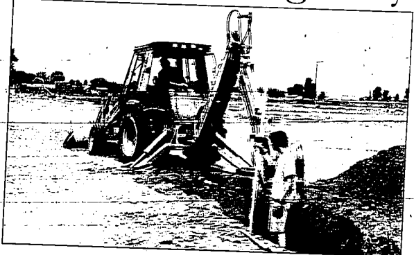
Kent Korb, operating the backhoe, and Greg Jones, of Gary W. Jones Construction in Burley, dig the footings for the new United Electric Co-op building in Heyburn. With a shovel and a laser level, Jones makes sure the trench is of uniform depth. The building, at 1330 21st St., should be completed by mid-December.
