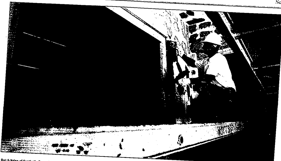
Butch Nolan of Synthetic Dynamics applies a cement coat to the dialysis center under construction near Pole Line Road in Twin Falls, a job site of general contractor Starr Corp. Nolan says having construction workers certified would benefit consumers.
