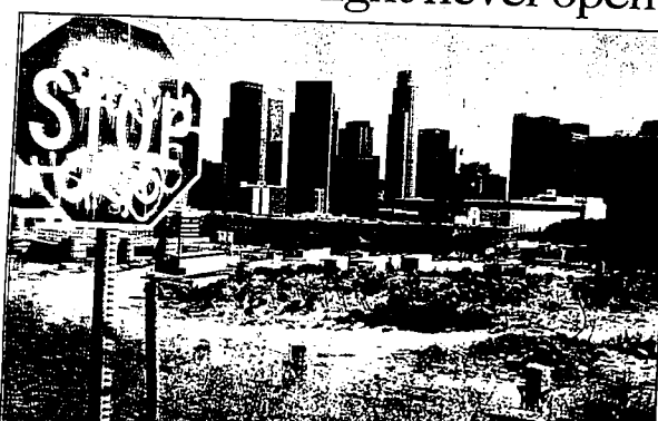
The 35-acre site of the Belmont Learning Center in downtown Los Angeles is reportedly the nation's costliest high school. Toxic gas leaks plague the half-completed site, and threats of contractor lawsuits loom over the school district.
