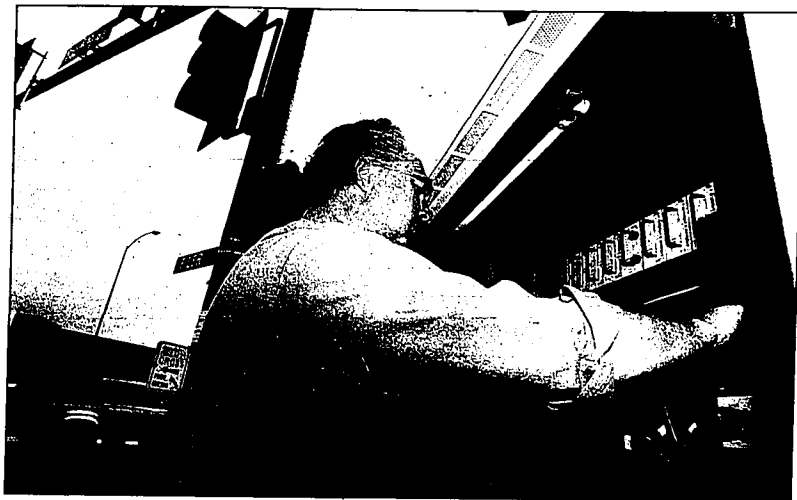
Assistant City Engineer Rod Mathis checks the lining on a traffic light at the intersection of Blue Lakes Blvd. and Filer Ave. When a new centralized system becomes fully operational, computers in City Hall will be able to count the cars at all the intersections in town.
