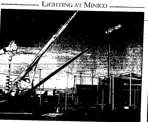
Bonneville Power Administration workers adjust a light pole at Minico's Warburton Field in Rupert Tuesday. By noon, the crew had set two of the eight poles. For more on the improvements at Minico High School's baseball diamond, see page D2.
