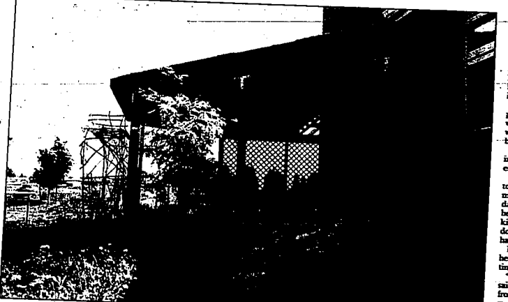
When building the patio, Bokma wanted a wood look, but didn't want the hassle. The patio is shaded by wood, and the floor is protected by another roof.
