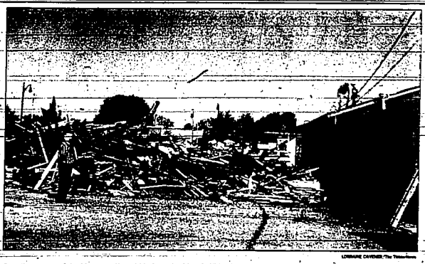
Standing on a roof, looking over the rubble from the Rios de Vida church, Bob West and Dave West, far right, inspect the Rupert Red Cross building roof for possible damage from the Aug. 21 fire which razed the church. The Red Cross building is next door to the church. Red Cross board member George Falkner stands on the ground and watches the inspection.
