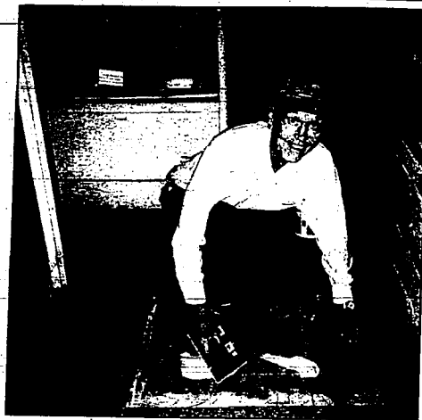
Above, Norman Dayley lays new tile in the general store at the Cassia County Historical Museum. Dayley's effort followed his restoration of hospital chairs at the museum. Below, Weldon Beck gathered children from his neighborhood to help chip old tile off the floor of the Cassia County Historical Museum's general store. The group is, from left to right, front row: Kaci Carpenter, Koby Carpenter, Kord Carpenter and Kade Carpenter; and back row: Sam Barress and Beck. The Cassia County Historical Society's annual membership dinner begins at 6 p.m. on Thursday at the Cassia County Historical Museum. Tickets for the dinner are $11 and reservations should be made before Friday. Annual dues are $8.50 for an individual or $12.50 for a family. For more information or reservations, call the museum at 678-7172.
