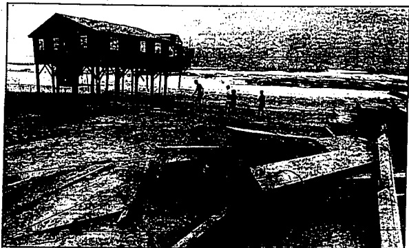
People walk past the remains of a house in Rodanthe, N.C., Friday, that was destroyed by Hurricane Dennis. Residents of Hatteras Island who were evacuated for the storm were allowed back to the island.
