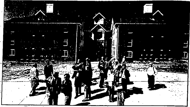
Members of the Olympic Coordination Committee and others tour the new student housing complex under construction at the University of Utah in Salt Lake City. The site will serve as the Olympic Village for the 2002 Winter Games.
