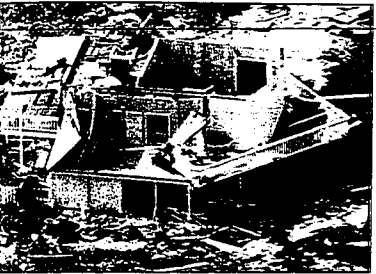
A destroyed home with its roof tipped off on the Grand Abaco Islands shows the results of Hurricane Floyd, Wednesday. Floyd struck the Bahamas on Tuesday with winds estimated at more than 110 mph.
