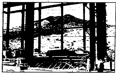
A Costa Rican power plant designed by Hailey's POWER Engineers is nearing startup. POWER also is managing construction at the geothermal plant site.
