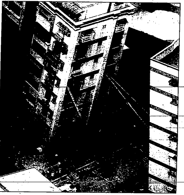
Steel beams prop up this apartment building Wednesday in Taipei, Taiwan. Many of the capital city's buildings just leaned over when the earthquake struck Tuesday.
