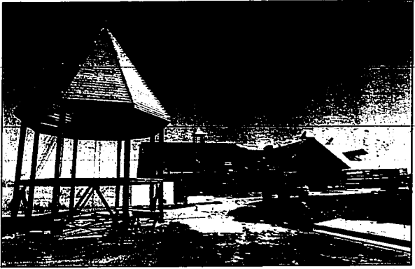
A cupola awaits placement atop the administration building of the new Fayette County Detention Center in Lexington, Ky. Designed to look like a typical stallion barn, the building will provide the base for a $71 million facility built to house up to 1,200 inmates.
