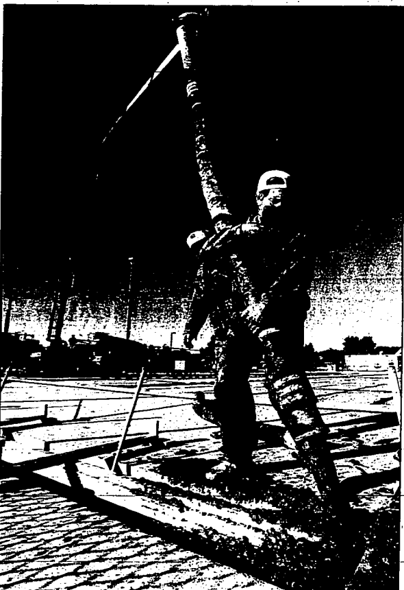
Gene Rine works with a concrete hose as cement is pumped into a footing that will secure the inflatable cover for the city pool. With construction done and the bubble ordered, officials plan to reopen the pool to the public this winter.
