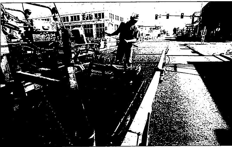
Bob Ryan checks the depth of the new asphalt on Main Street in Jerome. The project is nearing completion and officials hope to be done in time for the city's grand opening celebration for the downtown Saturday.
