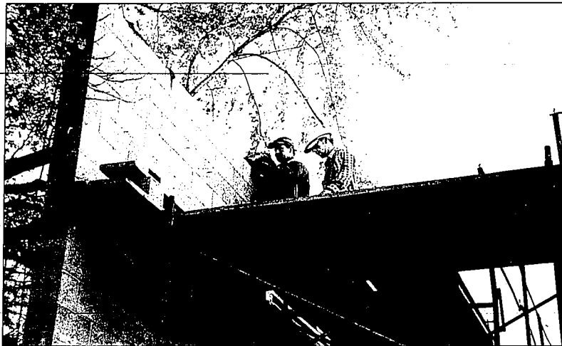
Willie McKinney, left, and Chris Braun pour grout for the new Towne Centre complex on Twin Falls' Blue Lakes Boulevard North. The complex will be ready to be occupied Dec. 1, its landlord said.
